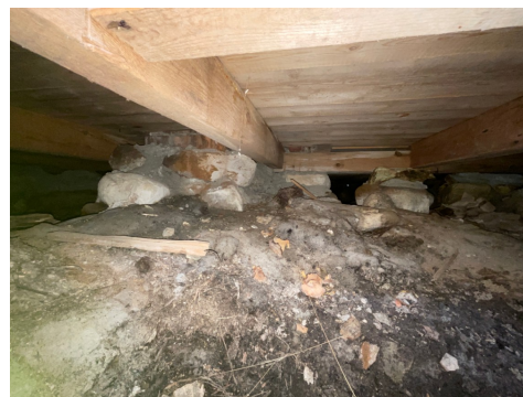
Fundament teglsteinspipe
