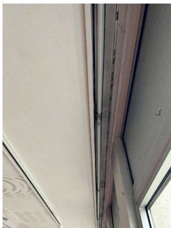
Eldre lysarmaturer langs vindusfelt i 2. et
