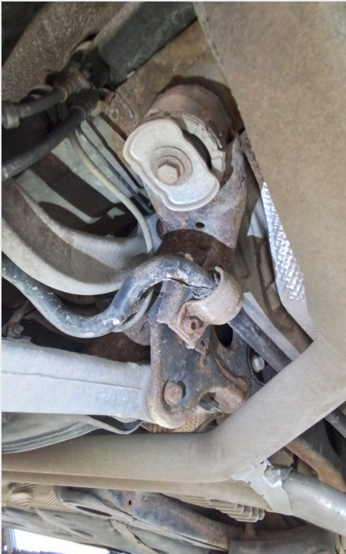
2.2 Noe rust travers bak
