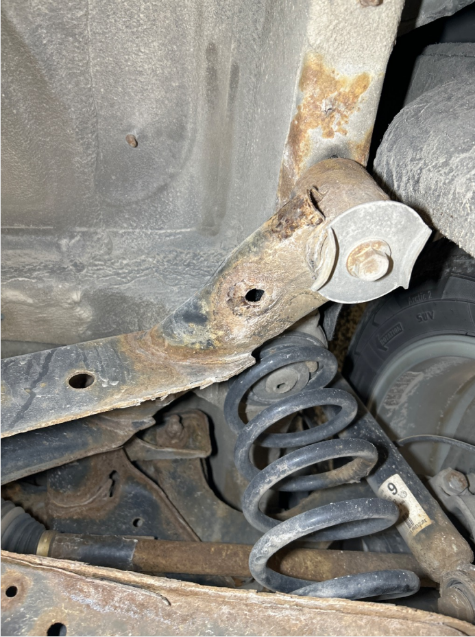
2.14 Rust finnes, travers bak
