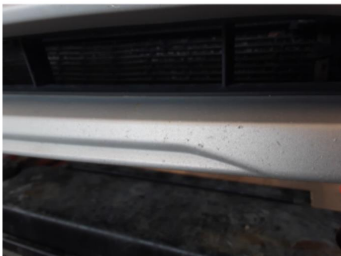
1.1 Noe steinsprut i front.
