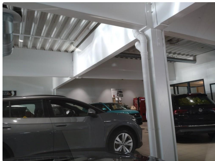
1.9 Steinsprut utenfor synsfelt
