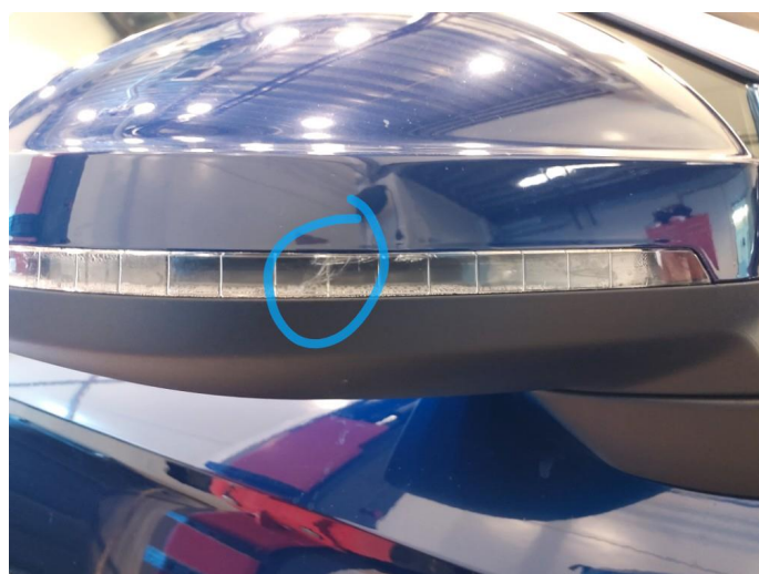
2.1 Krakelering i plast
