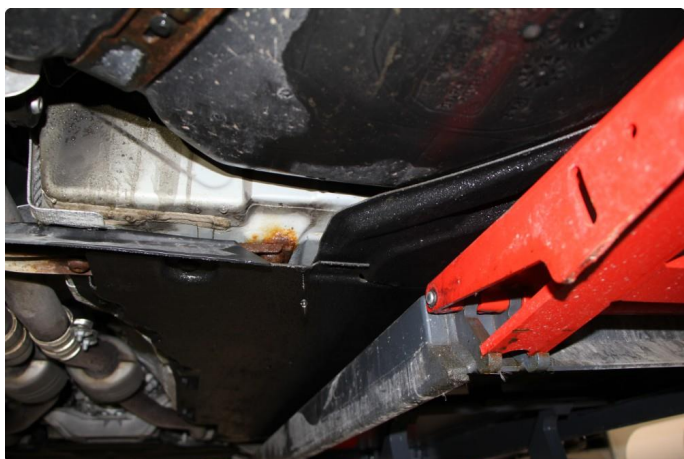
1.2 Noe rust under bil
