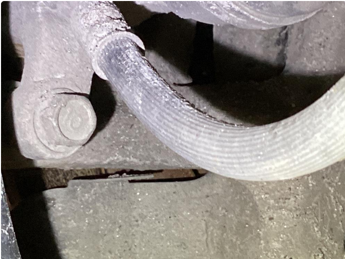
1.1 Mer enn 25% rust
