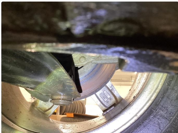
2.1 Mer enn 25% rust
