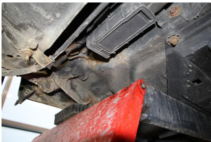
1.2 Litt rust i chassiss
