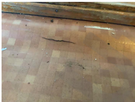
Skadet vinylbelegg.
