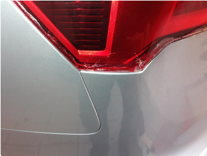
2.1 Noe krakelering i plast
