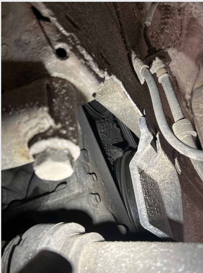
5.11 Mye svetting motor, lekkasje?
