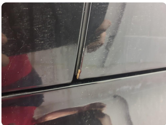
2.5 Rust i fals
