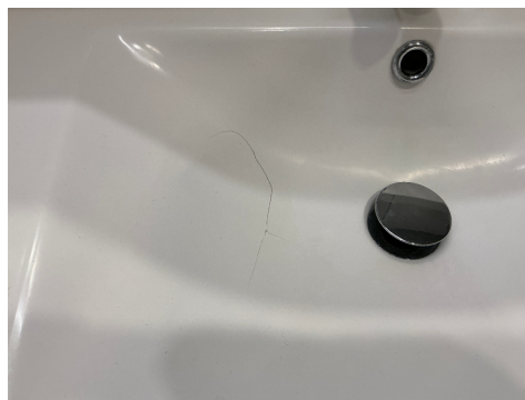
Sprekk i servant
