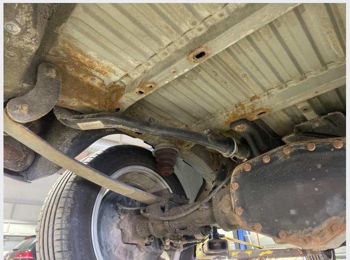
2.2 Litt overflate rust
