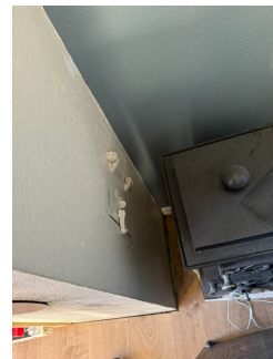
Sotluke i pipe, manglende ubrennbar plate under.
