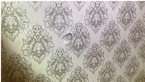
Hull i vegg.
