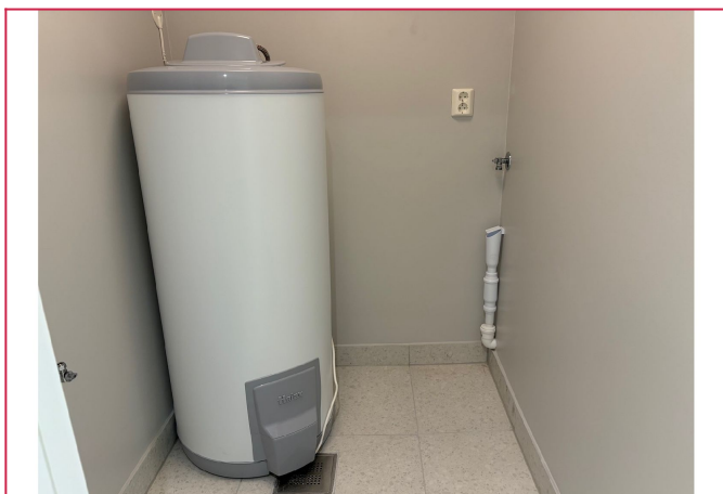
Opplegg for vaskemaskin
