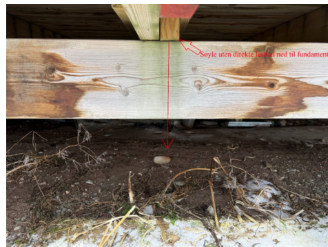
Mangler fundament
