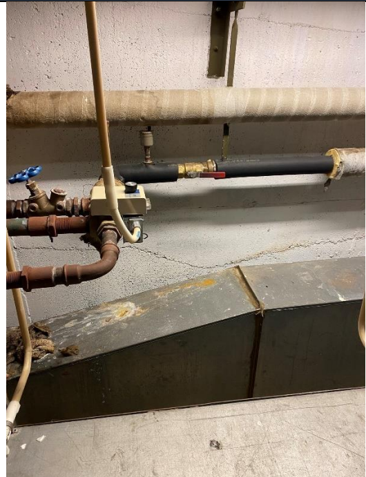
Plassering: Vent.rom over gymsal Materialtype: Cellegummi
