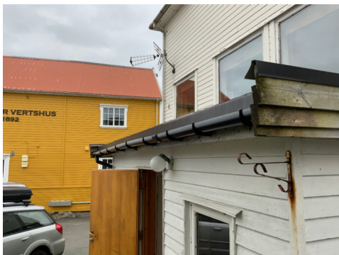
Deformerte renner
