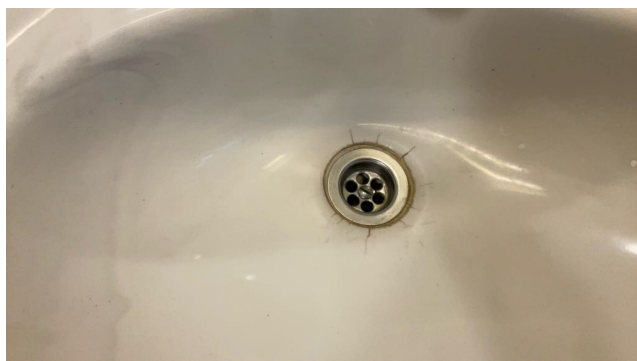
Riss i servant.
