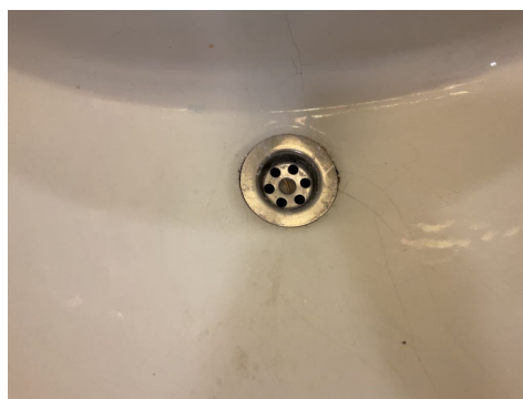
Krakelering i servant
