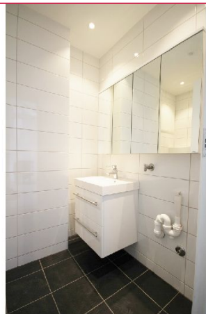
Opplegg for vaskemaskin.
