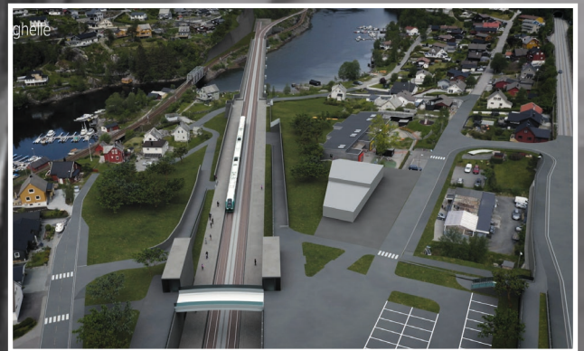
New Railway station at Stanghelle
