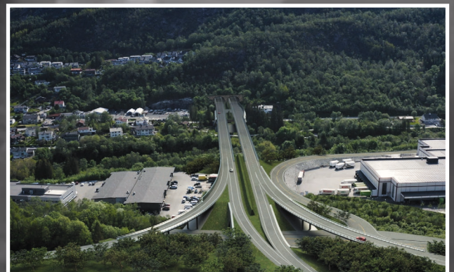
Double tube road tunnel Arna - Trengereid
