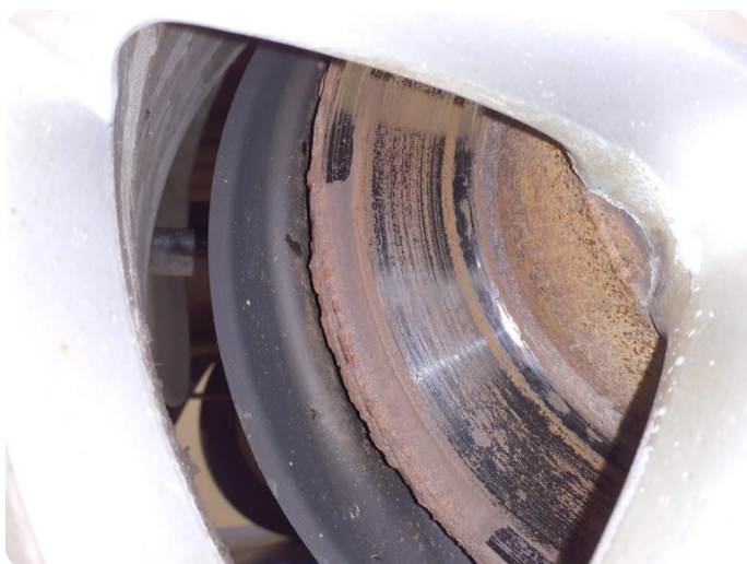
6.1 Slitte/stor slitekant Tillegg rust bremses bak
