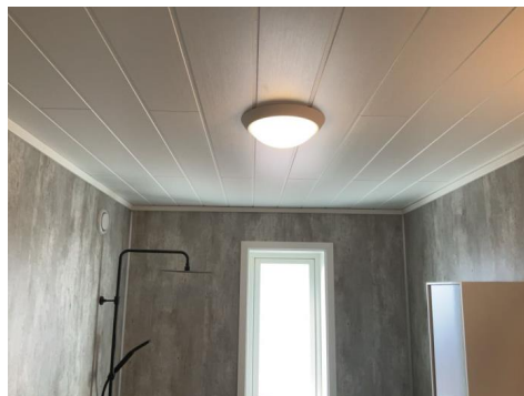
Takpanel i taket.
