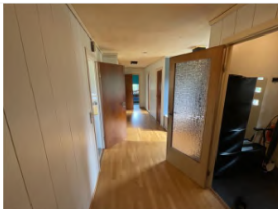
Overflater i gang
