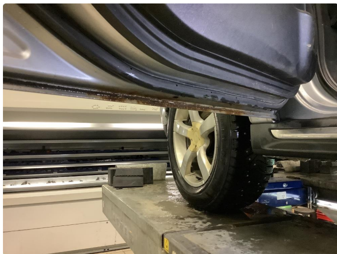
1.2 Rust i fals
