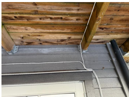
Bjelkesko montert i panel
