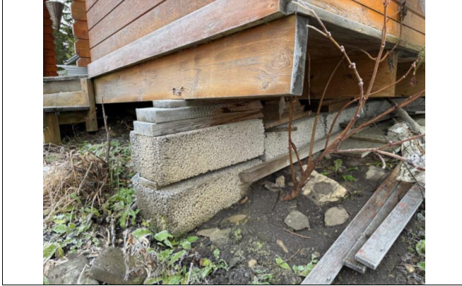
Enkel fundamentering under bassenghus
