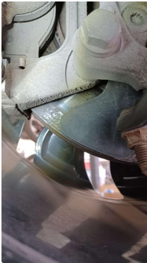
2.1 Mer enn 25% rust
