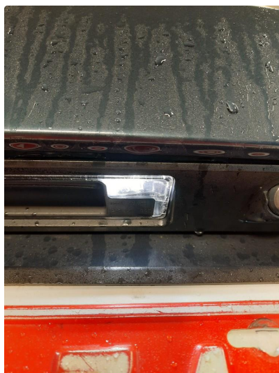
2.1 Krakelering i plast
